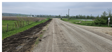
Grant Wood Trail construction alongside Oxley Rd to Secrist Rd.
