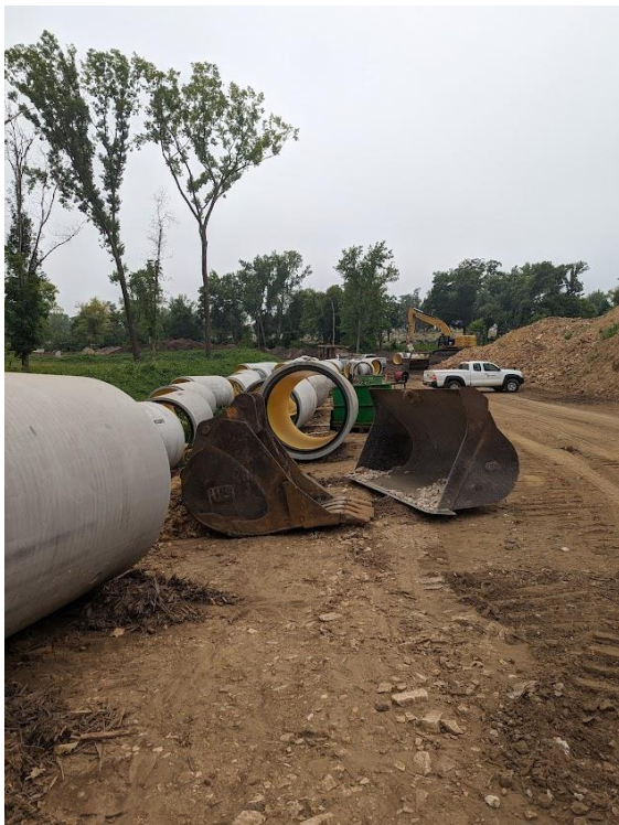
Indian Creek Trunk Sewer Project
