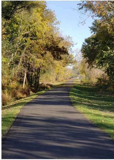
Marion paved the last section of crushed rock trail west of the new bridges over Indian Creek and Marion Boulevard.
